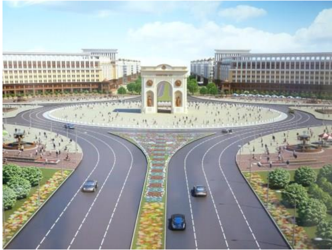
Fig. 4 A proposal in the master plan where the human scale is lost. These wide free-flow designs create situations in which it is almost impossible to safely integrate cycling.
