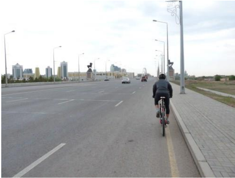
Fig. 6 With such wide roads it is easy to create a cycle track by taking away one lane for motorized traffic.
