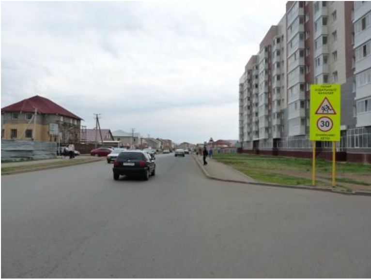
Fig. 14 Traffic calming is a good idea, but without the proper design speeds will not go down. This road is clearly much too wide for to entice drivers to slow down.
