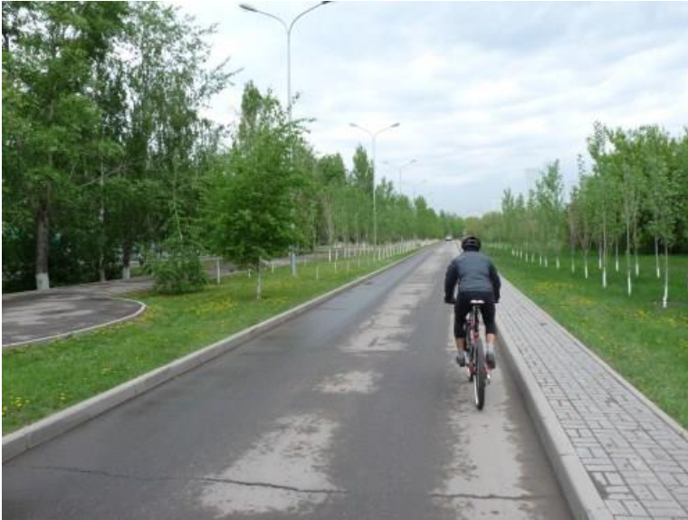
Fig. 9 Even in parks car-accessibility and road infrastructure is dominating. But it won't be difficult to construct cycle tracks throughout green areas such as these.
